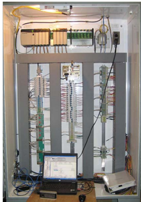
Figure 12. The hydraulics upgrade included all new PLC control hardware and software which were tested in advance at a Valmet workshop.
